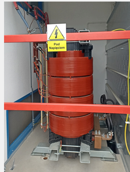
TRANSFORMER: 1250KVA 15,75/0,39 kV PHOTO: ZPUE S.A.
